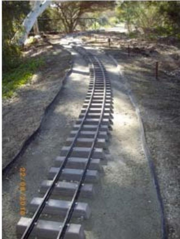
The following Friday again saw rail and sleeper wagons loaded ready to go, along with additional tek screws etc being sourced, with all in readiness to go for the final push on the Saturday. Again, a crew set about assembling the final sections of track to be installed, while the roadbed levels were finished off. Track was being slid into place just prior to morning tea, with welding of joints following not long after.
